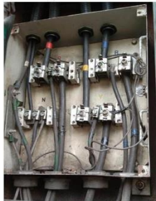
Allen-Bolt (Type-I) old RCF design
