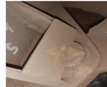
Fig-Welding of APD with Pin & Brake cylinder body
