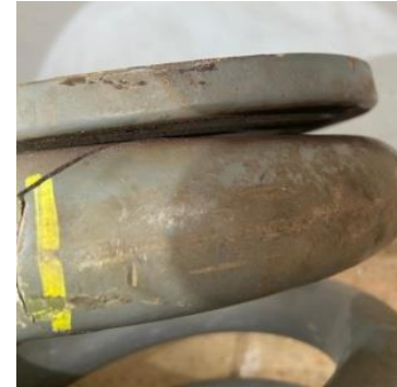
4 th Case Rly- MMCT-GNC Location: Bottom This happened 2nd time, earlier spring was broken at the same location as mentioned in 2nd case. This spring was failed within 7 days after replacement. Now bogie has been replaced.
