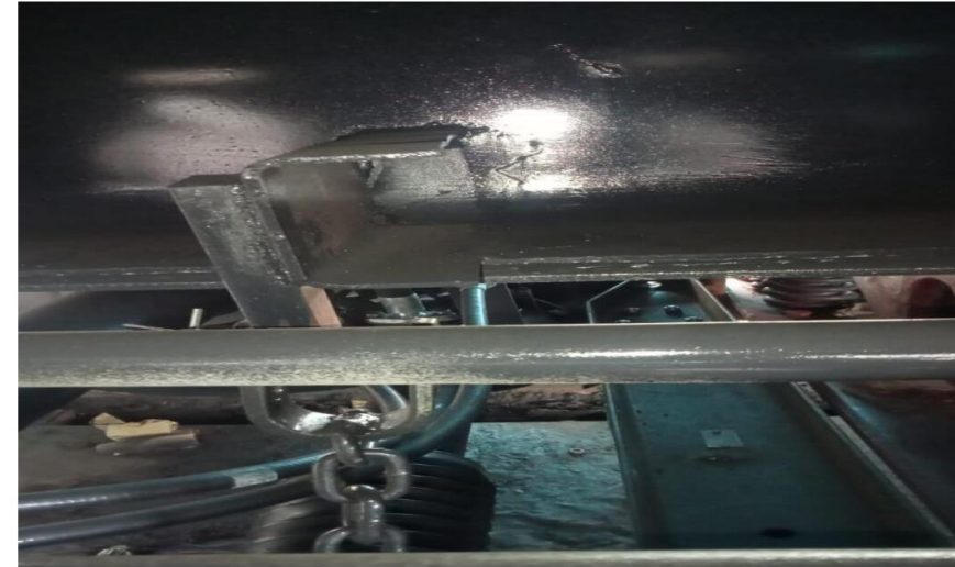
Fig 5- Safety Chain Welding- (Lap joint)
