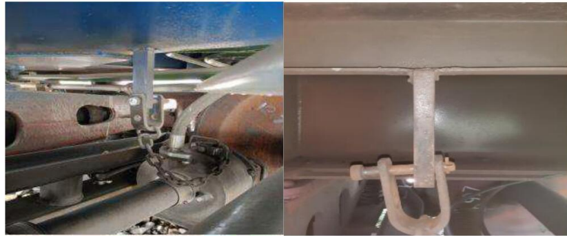
Fig 6- Safety Chain Welding- (Butt joint)
