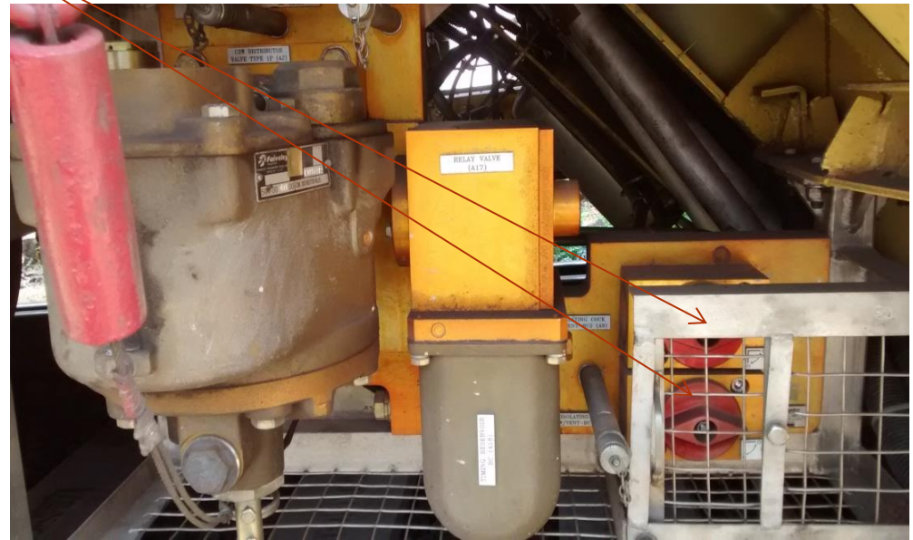
FTRIL CONTROL PANEL
